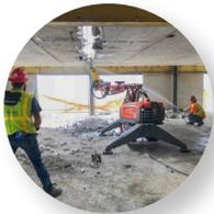
Our team designed a multipurpose excavator based unit capable of remotely entering the dome with a long front boom capable of reaching 60' with a light weight bucket and cement vacuum suction attachment.
